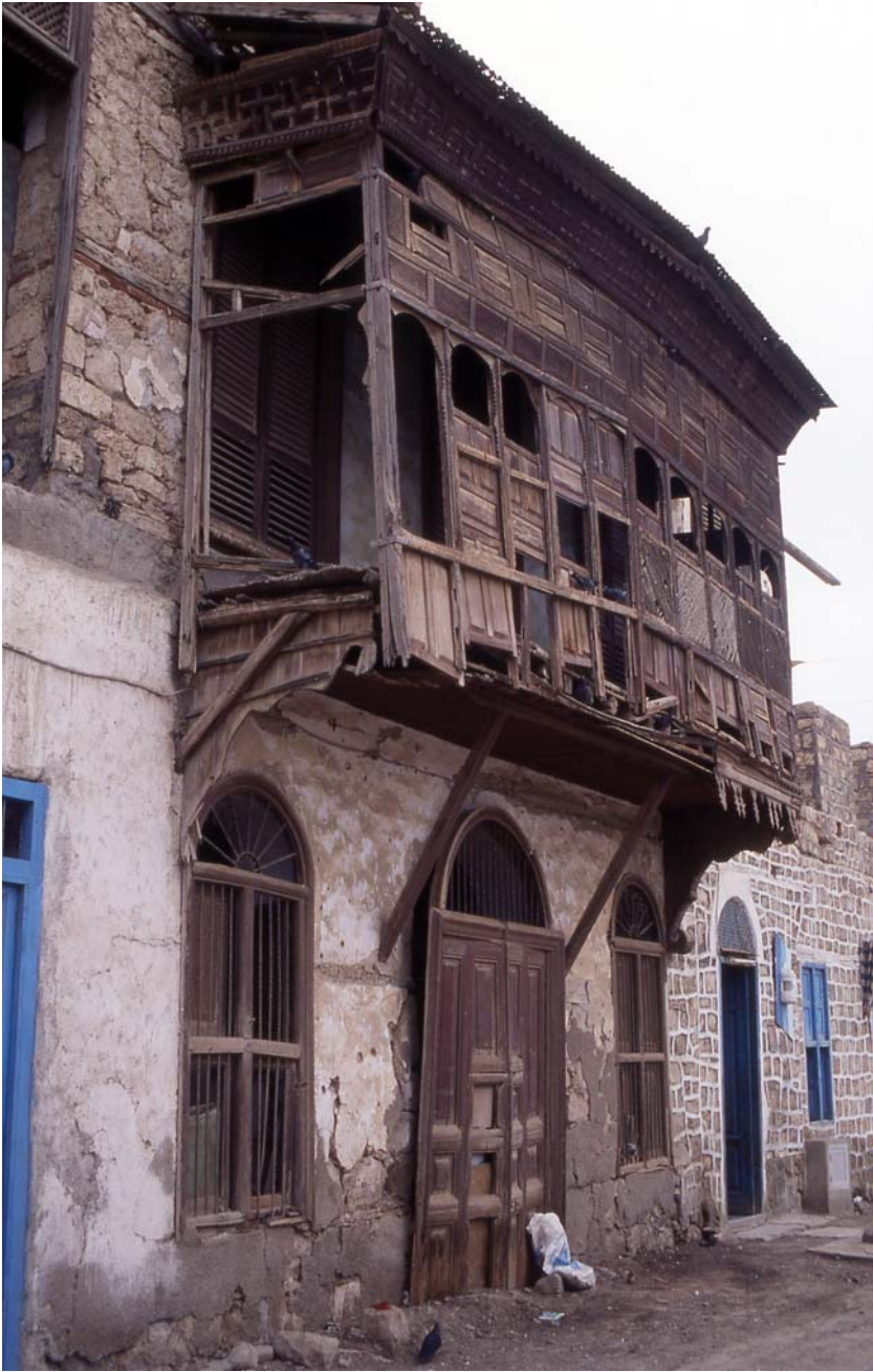
Figure 5. Bā Hamdūn house, Massawa, Eritrea. Photograph by Dennis Rodwell, © Dennis Rodwell.
